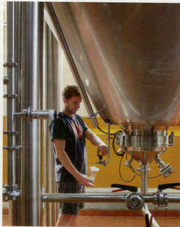
ON TAP Workers can sample beer via spigots at the tapered base of each tank (left). Each 40-foot-tall tank has a 300-barrel capacity, and is accessed by way of a staircase on the southeast wall (right) that leads up to a steel-grate catwalk. Employees can then add anti-clouding agents and other ingredients to each vat.
